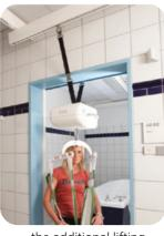
... the additional lifting strap must be linked to the track in the adjacent room..
